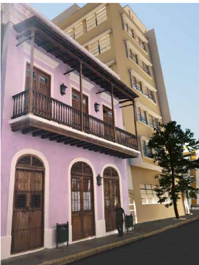
Exterior | View from Cruz Street
