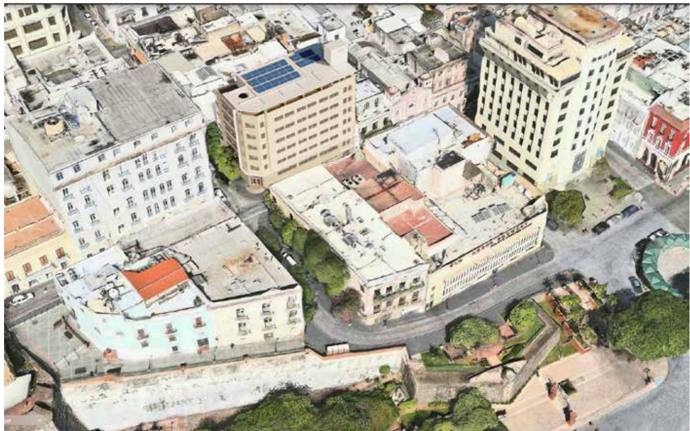
Exterior | South aerial view
