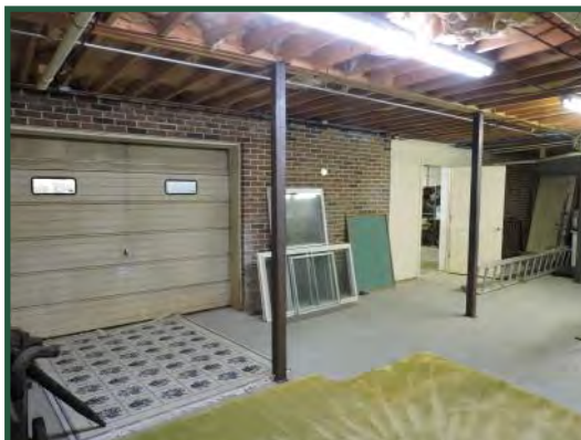
Basement General Storage
