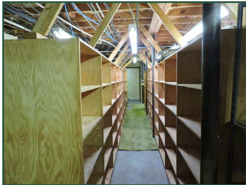
Storage and exposed plumbing
