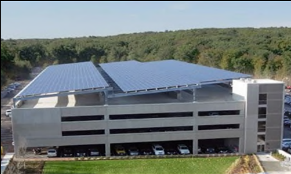
A 684-kW installation at Staples' HQ
