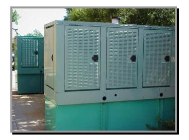
In addition to our DC power plants, our entire facility is backed-up by two standalone 150KW diesel generators to protect against any external power outages.
