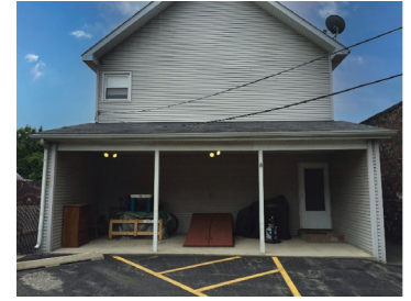
Rear View (Unit C Entry)
