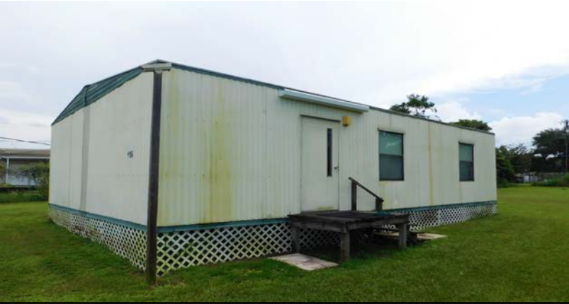
Building 1 - Double Wide Office
