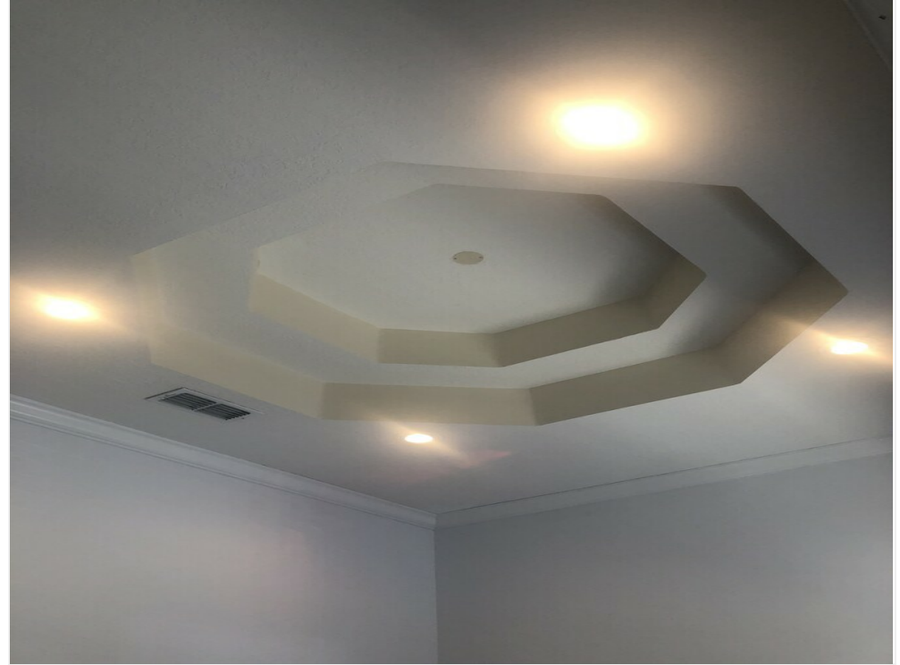
E - Reception Vaulted Tray Ceiling I
