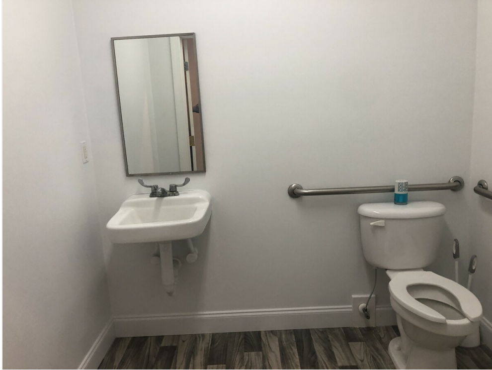
P - ADA Compliant Restroom With New Floors II
