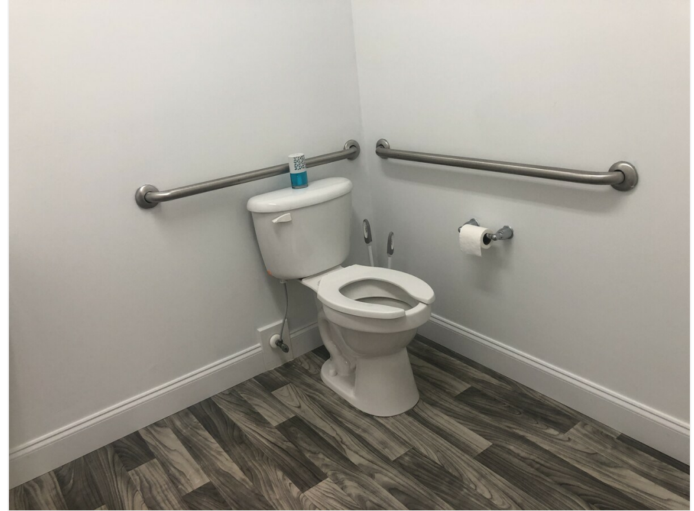
Q - ADA Compliant Restroom With New Floors
