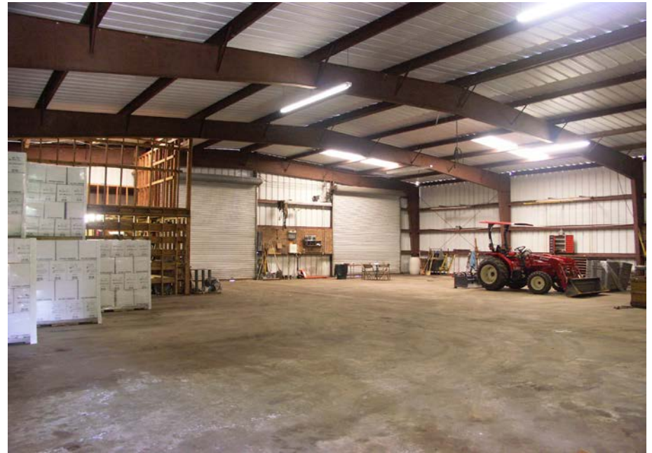
Metal building with steel construction 2 - 12" roll up doors
