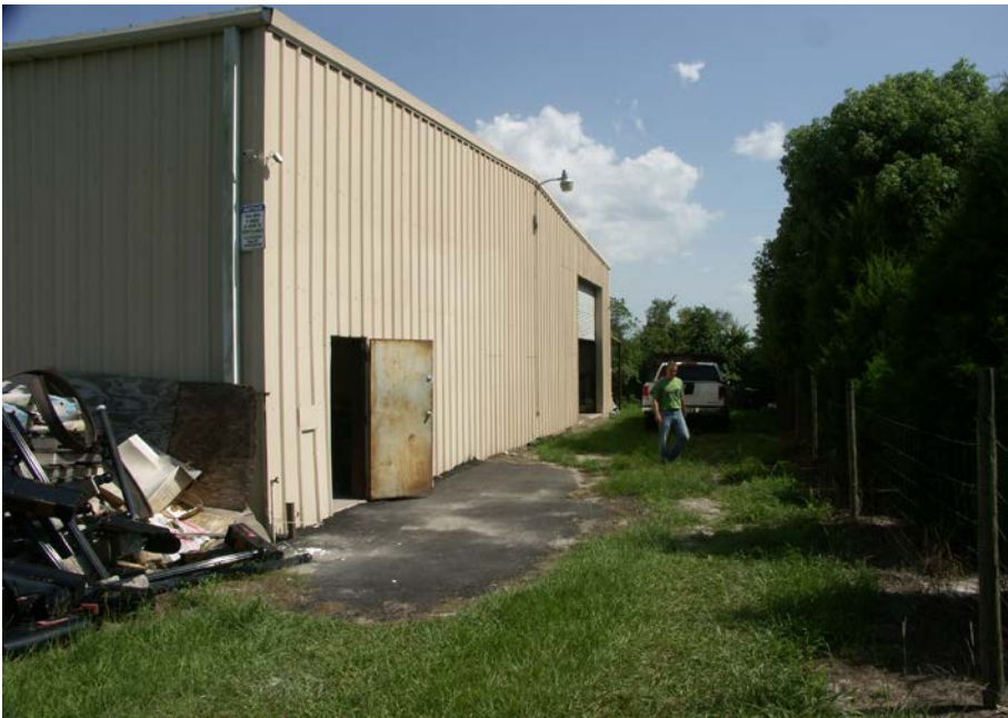
Side view with security camera
