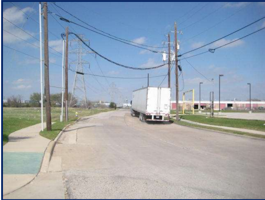
View of frontage along Wire Way Drive facing north with the nightclub property on the left.
