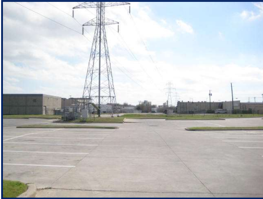
View of an overhead power transmission line extending north from Northwest Highway across 10557 Wire Way Drive parking lot.
