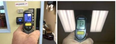
Air conditioning system was functional but it produced an improper temperature differential of less than 10 degrees. Acceptable temperature differential is 15 to 22 degrees. I recommend having the system serviced by a licensed air conditioning contractor to ensure proper and efficient operation. Heat Pump w/ Aux. or Emergency Heat.
