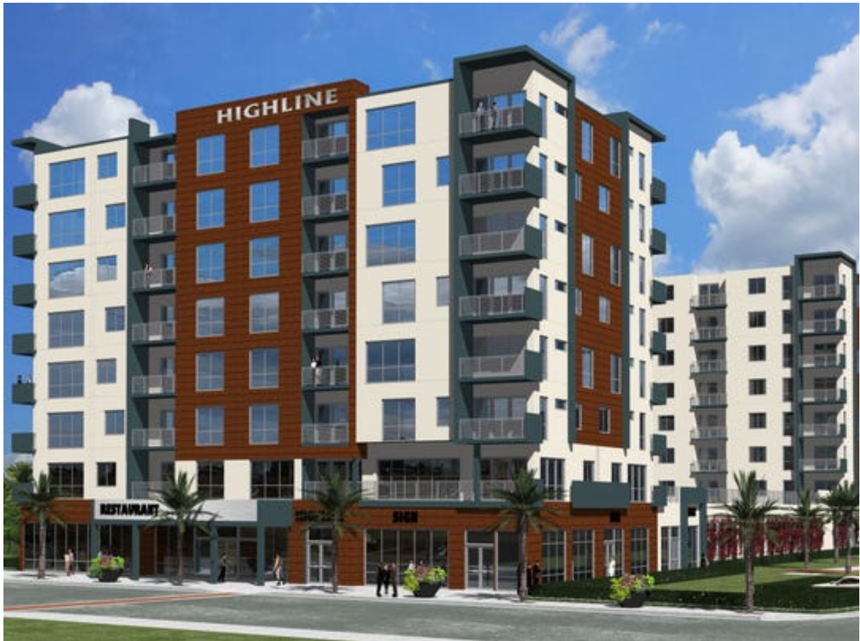
This artist's rendering depicts the eight-story Highline development, featuring 171 apartments at the former Melbourne High site on New Haven Avenue. (Photo: Courtesy of Caribeño Architectu)
