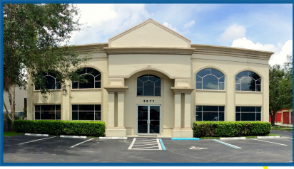
Building/Front Parking Area
