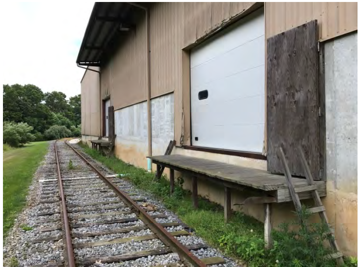
Rail Service And Loading Doors
