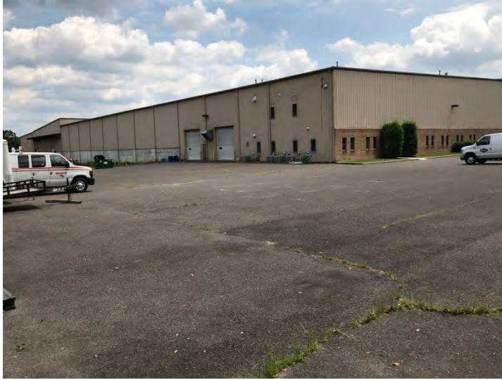
Northside Of The Warehouse
