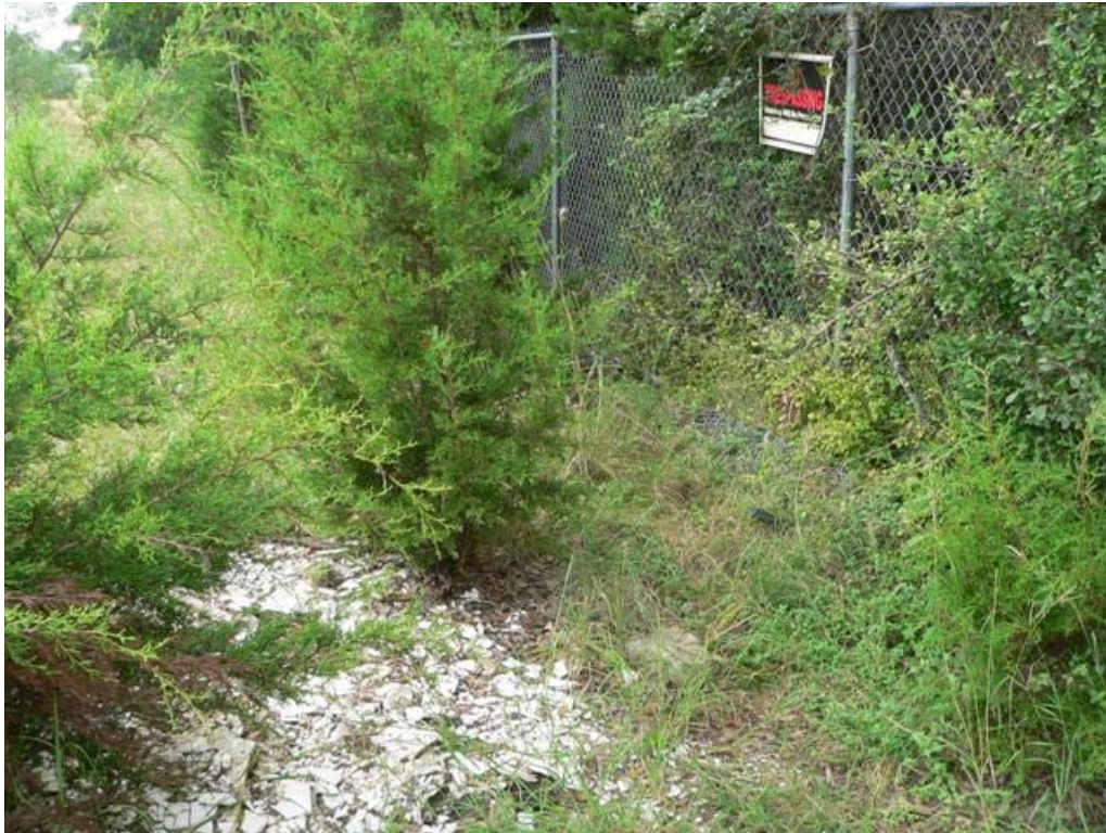
Photo No. 3: Limestone fragments and asphalt was visible at the surface on the Subject Property.
