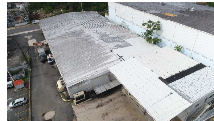
PHOTO: EXTERIOR (ROOF)
