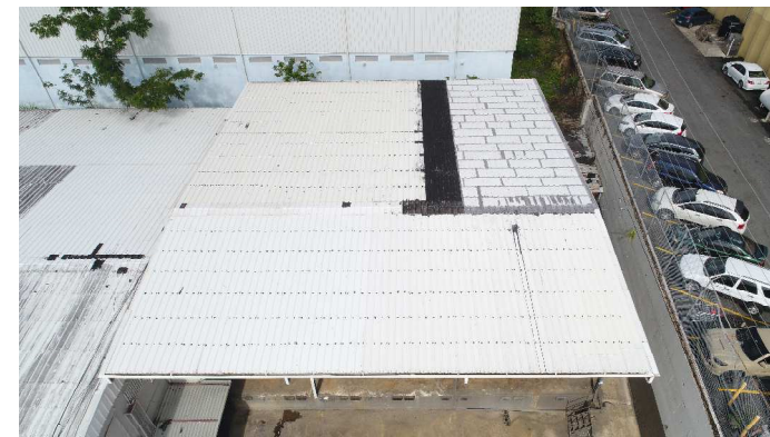
PHOTO: EXTERIOR (ROOF)
