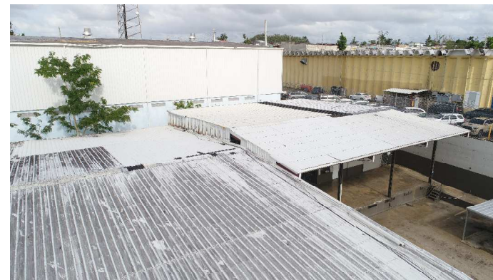
PHOTO: EXTERIOR (ROOF)
