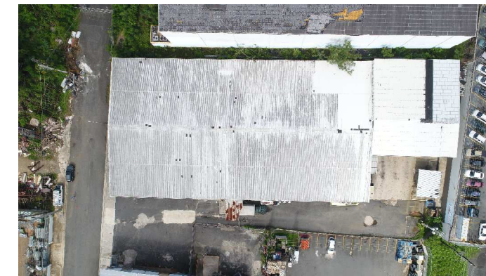
PHOTO: EXTERIOR (ROOF)
