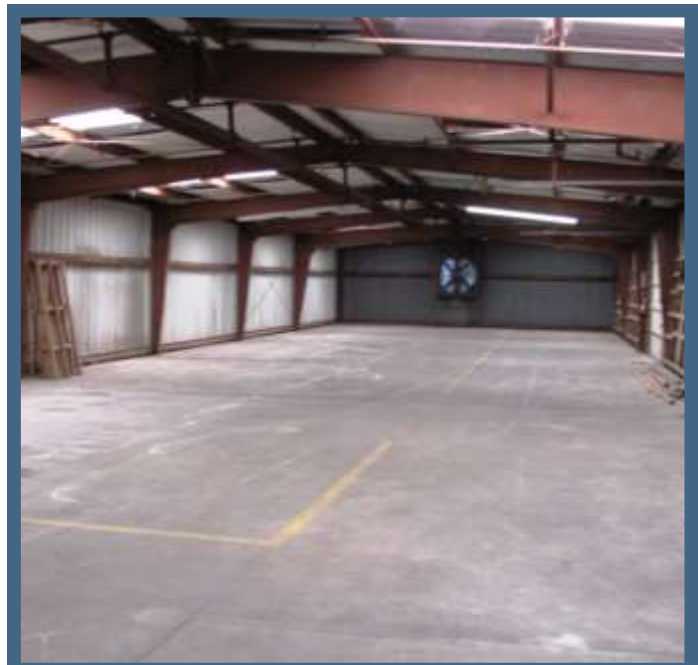
Second Bldg - No Columns
