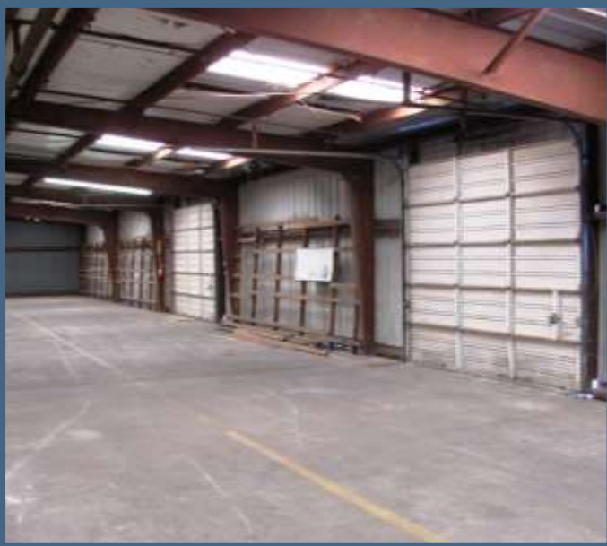
3 Large Overhead Doors
