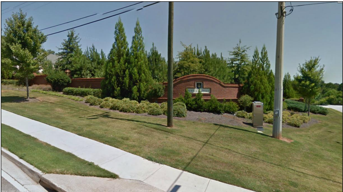
VIEW OF SUBJECT FROM CORNER
