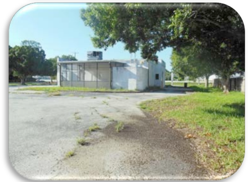
View from rear showing drive-thru
