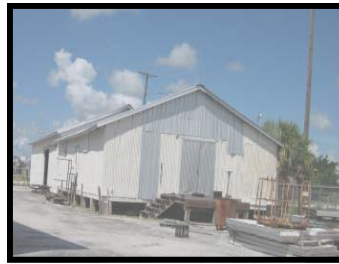
CB & Wood frame-metal roof -elec. Ramp, 30x100 Enclosed Storage (#12)
