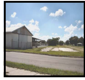
Area beside bldg. to left-former rail siding.
