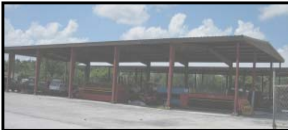
Buildings 10 & 11- Open storage 50x120' asphalt floor-no power 16' high 40x120-pole bldg.-metal roof- asphalt floor
