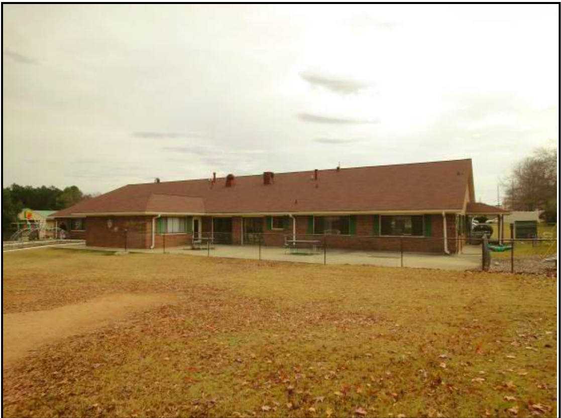
REAR VIEW OF SUBJECT
