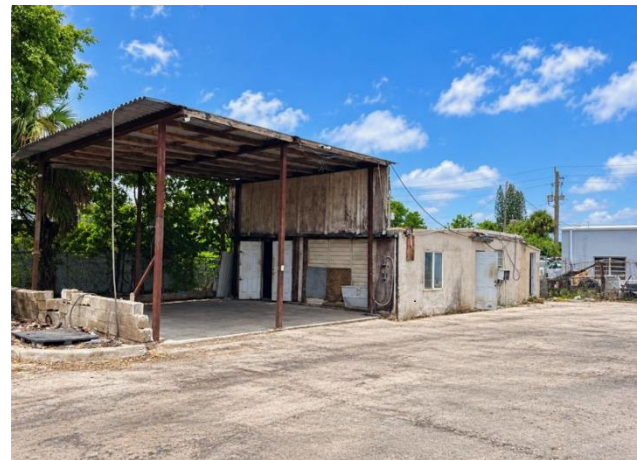
Small Bldg. & Overhang
