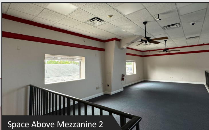
Stairs to Mezzanine 2
