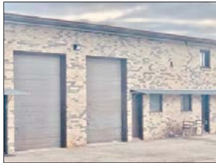
Dock High Doors C7 & C8
