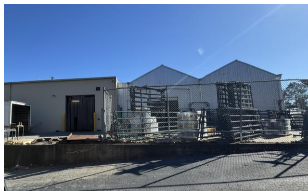
Roll up doors – Building & Garden Center
