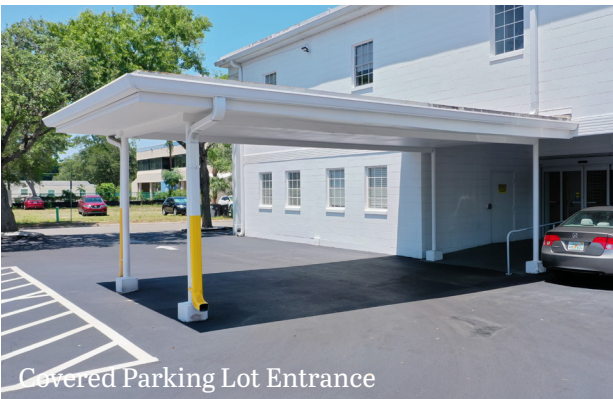
Parking Lot Entrance to Lobby
