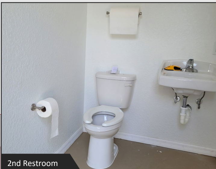
ADA Compliant Restroom
