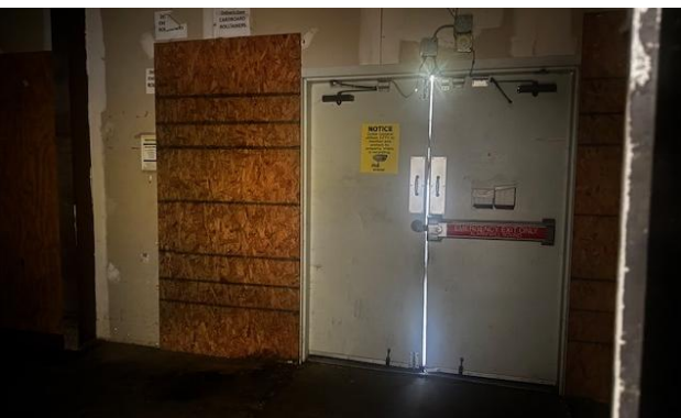
Warehouse at rear loading area
