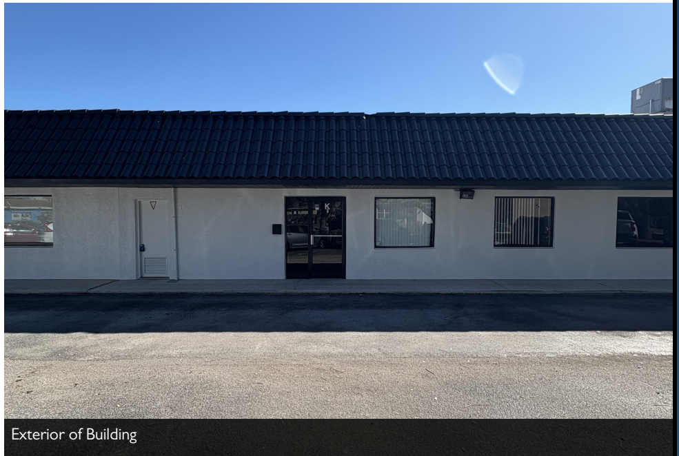
Exterior of Building
