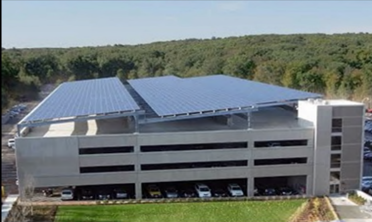
A 684-kW installation at Staples' HQ
