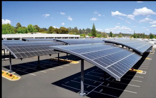
Solar Canopies for Parking Lots
