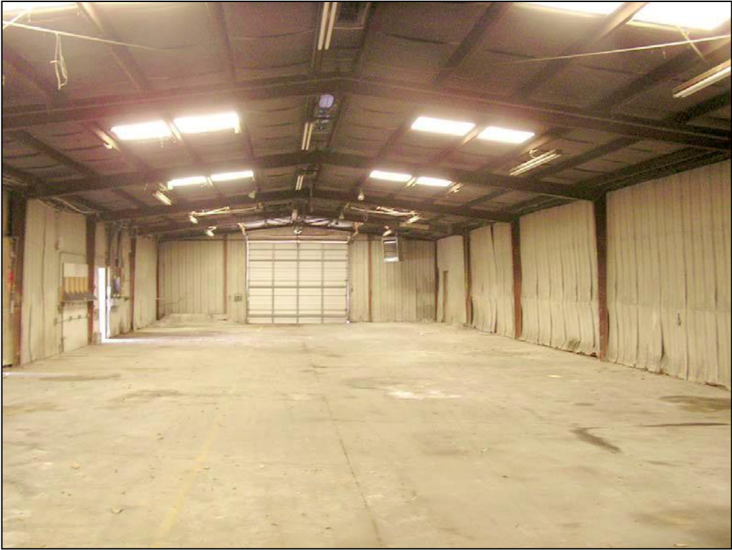
INTERIOR WAREHOUSE VIEW
