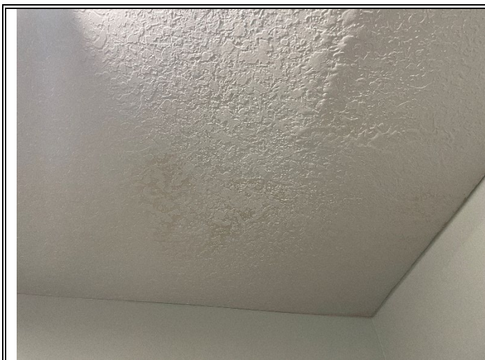
Photo 49: Water staining was observed on the ceiling below the air handler.
