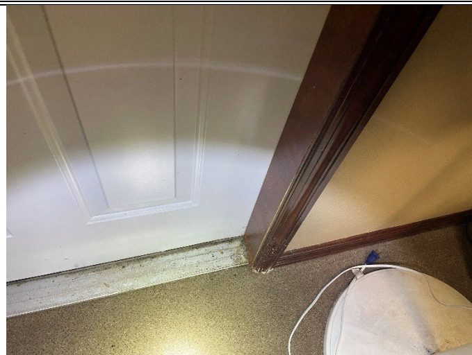
Photo 39: Water damage was observed at the base of the rear exit door trim.
