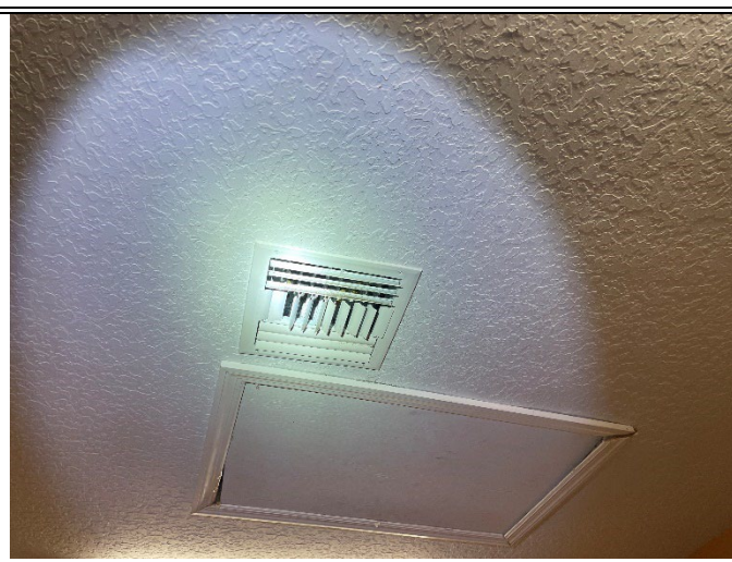
Photo 46: Visible suspect mold growth was observed on the supply vent next to the attic hatch.
