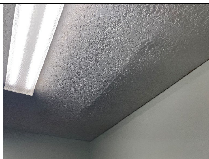
Photo 50: The ceiling was bowed downward below the air handler.
