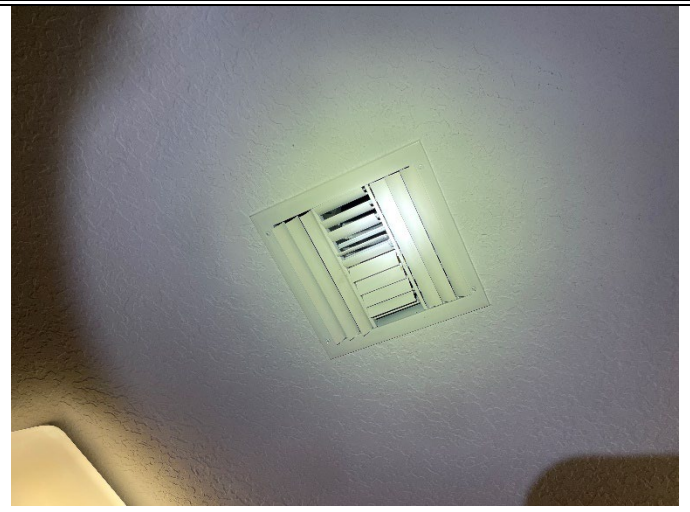
Photo 60: Slight visible suspect mold growth was observed on the supply vent.
