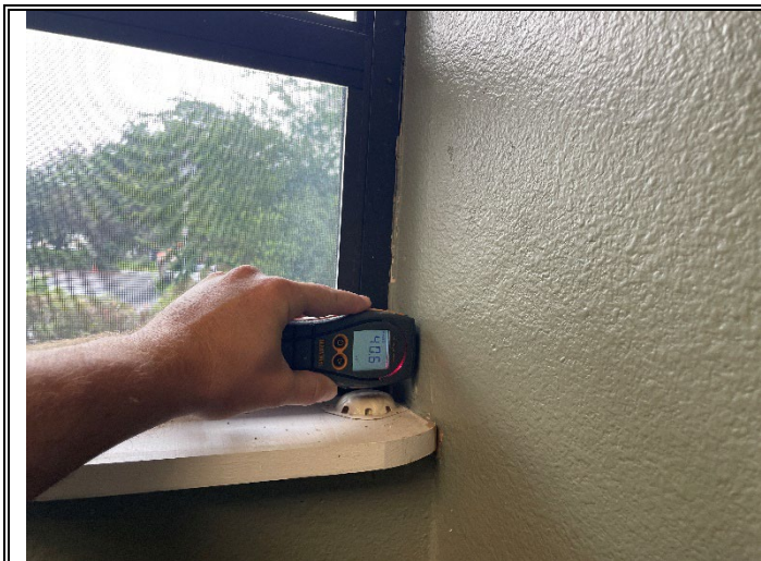
Photo 55: Elevated moisture was detected in the drywall below the break room window and rear wall.
