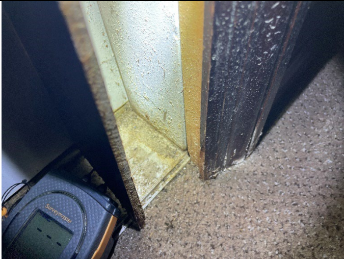
Photo 41: Visible suspect mold growth was observed at the base of the rear exit door frame behind the trim.
