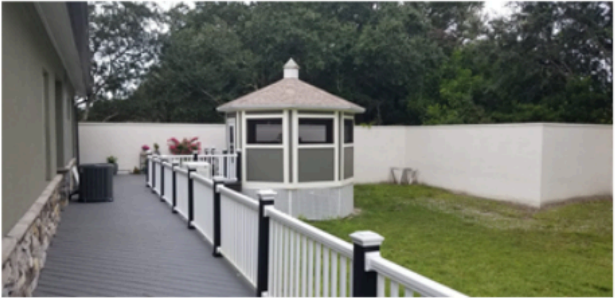
Side View of Two-Story Unit with Gazebo
