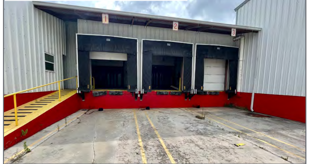
3 DOCK-HIGH DOORS ALONG WESTERN SIDE
