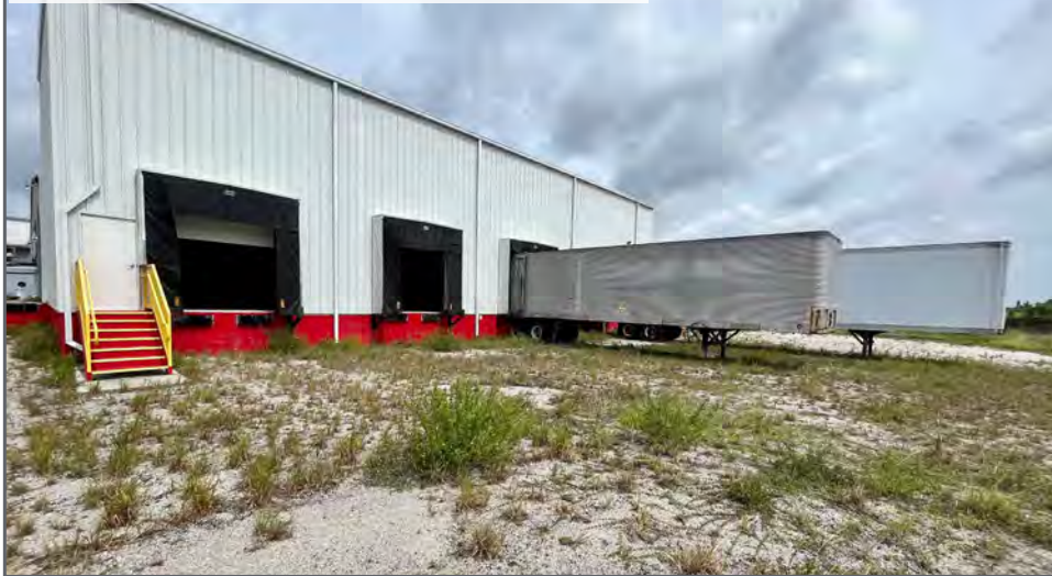
4 DOCK-HIGH DOORS ALONG EASTERN SIDE
