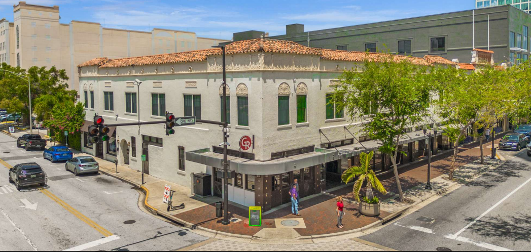
Corner of Orange Avenue & Washington Street
