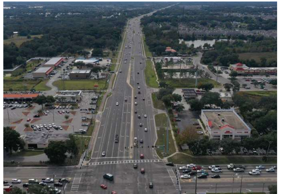
Aerial facing S
