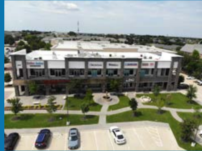
BUILDING B | 9244 PRESTMONT PL
