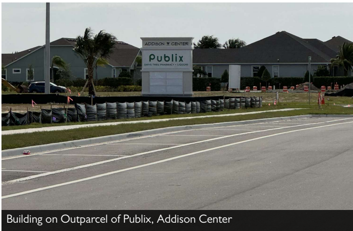
Construction to Begin Here
