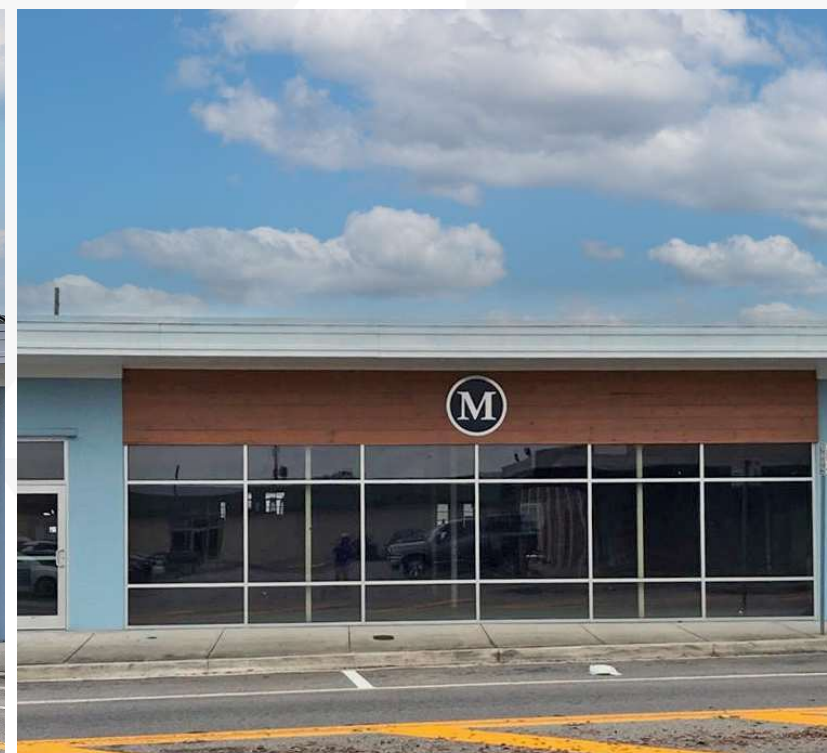
2010 North Orange Avenue
