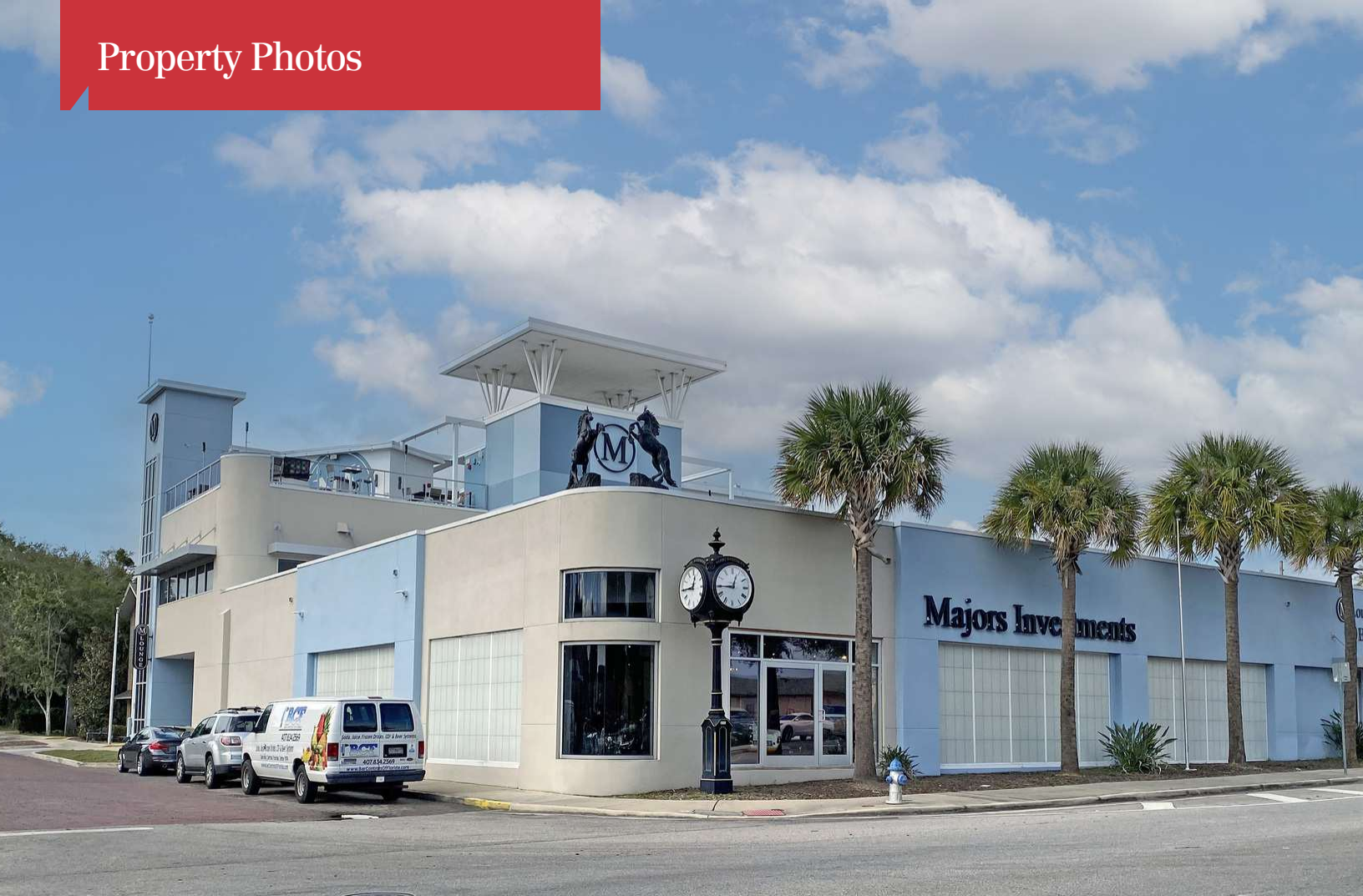
2000 North Orange Avenue
