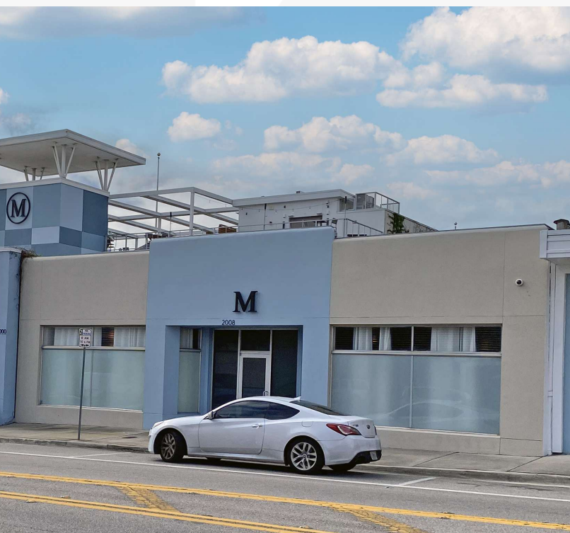
2008 North Orange Avenue
