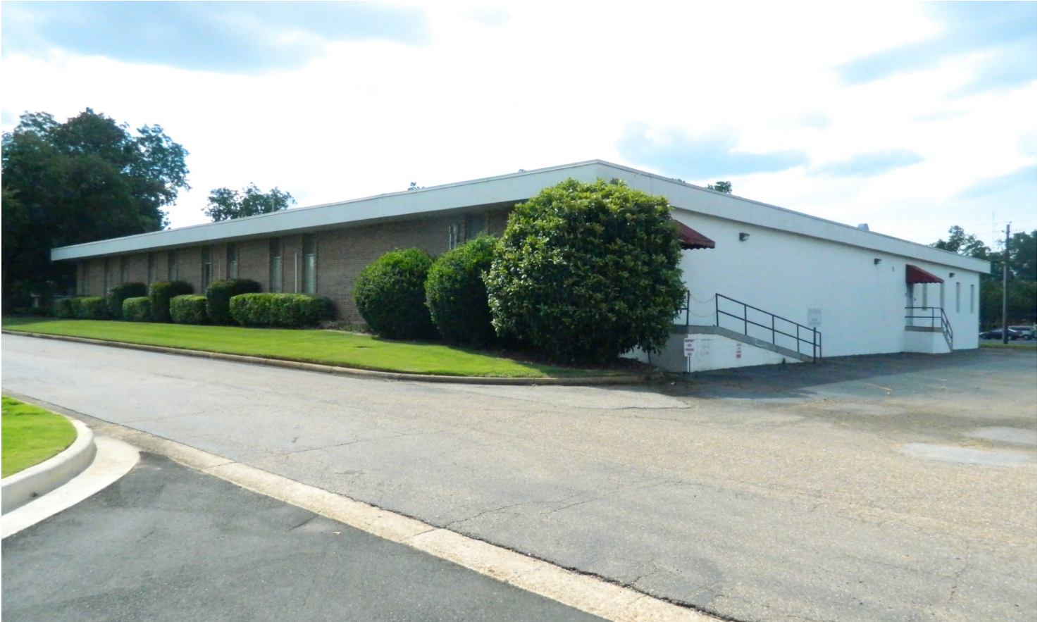
BUILDING I - BACK
