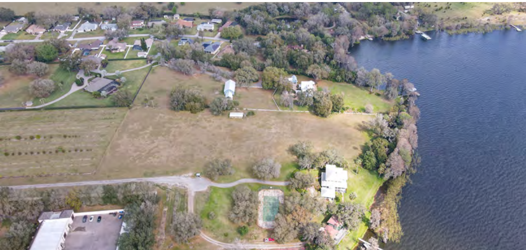
Aerial Facing North
