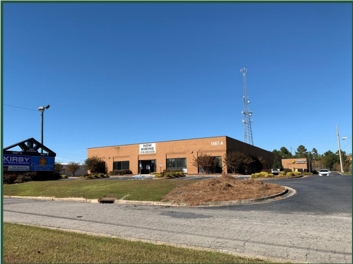
Building A Front
