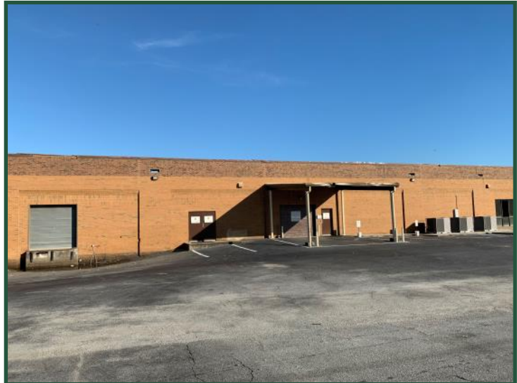
Building A Side with Roll-Up Door
