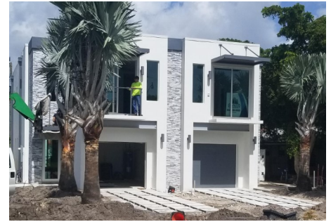
Medina Duplex New Construction and Site Work
