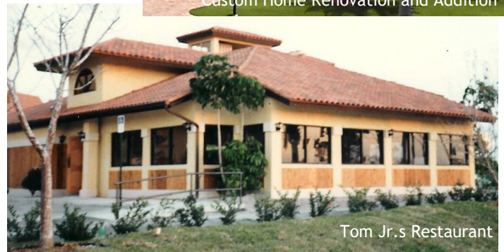
Custom Home Renovation and Addition
