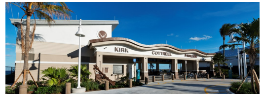
Kirk Cottrell Pavilion, City of Deerfield Beach , New Construction
