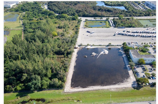
North Mass Transit Bus Parking Major Site Work
