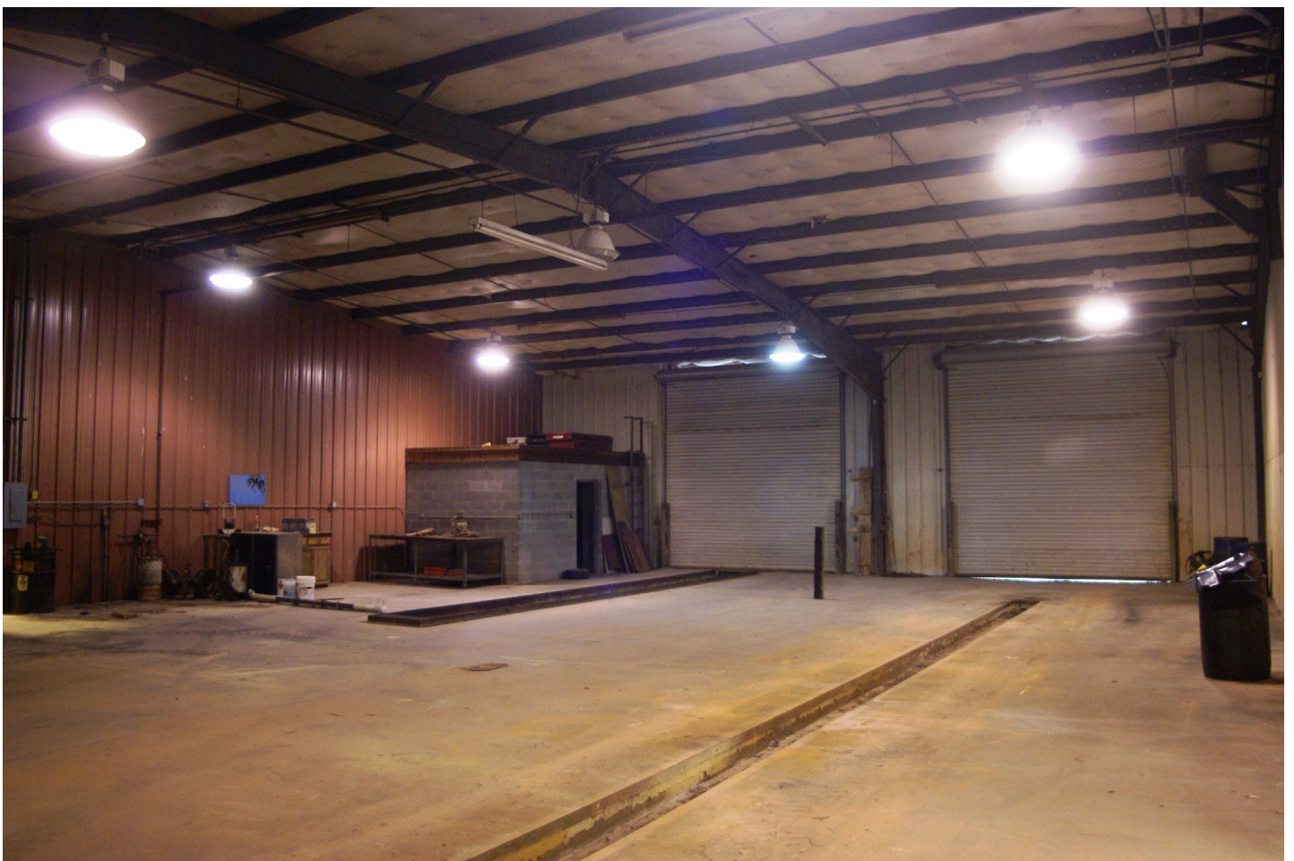
Bays 3 and 4 with grease pit and wash drain
