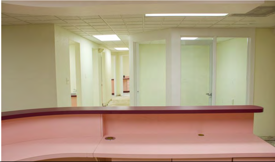
Alt. View - Reception Area Vanilla Shell - Flooring + Baseboards removed.
