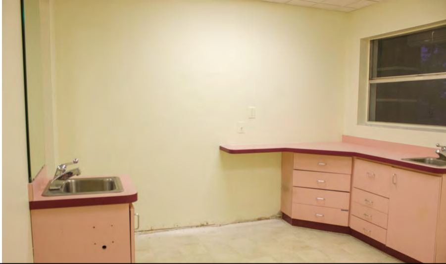
Exam Room 1 - Vanilla Shell - Flooring + Baseboards removed.
