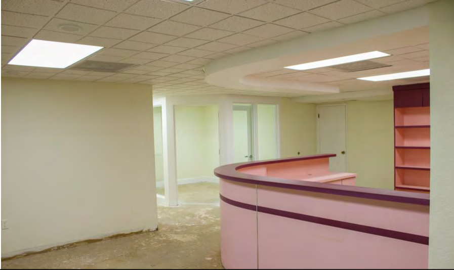
Reception Waiting Area - Vanilla Shell - Flooring + Baseboards removed.
