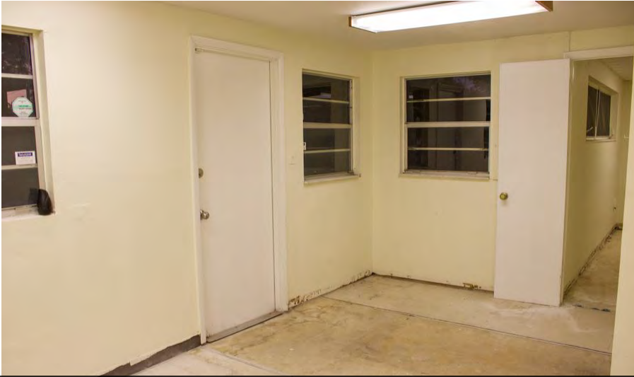
Back Office Area - Vanilla Shell - Flooring + Baseboards removed.
