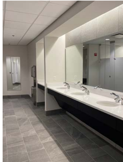
LOBBY MODERNIZATION Common Corridor & Restroom Upgrades
