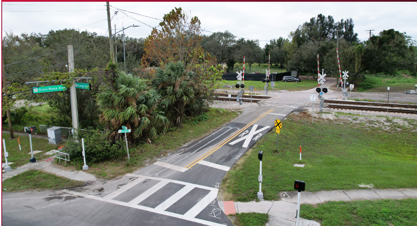
VIEW OF RAILROAD CROSSING IN-PLACE
