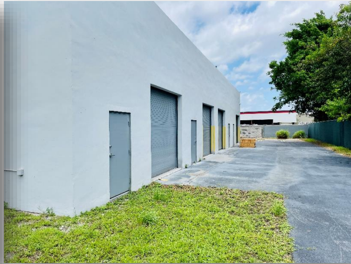
Rear Building 5 Grade Level Doors
