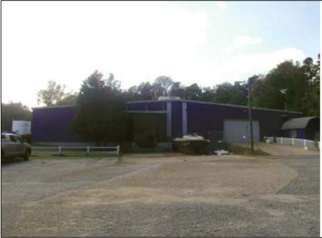
SIDE VIEW OF SUBJECT & LOADING DOCK
