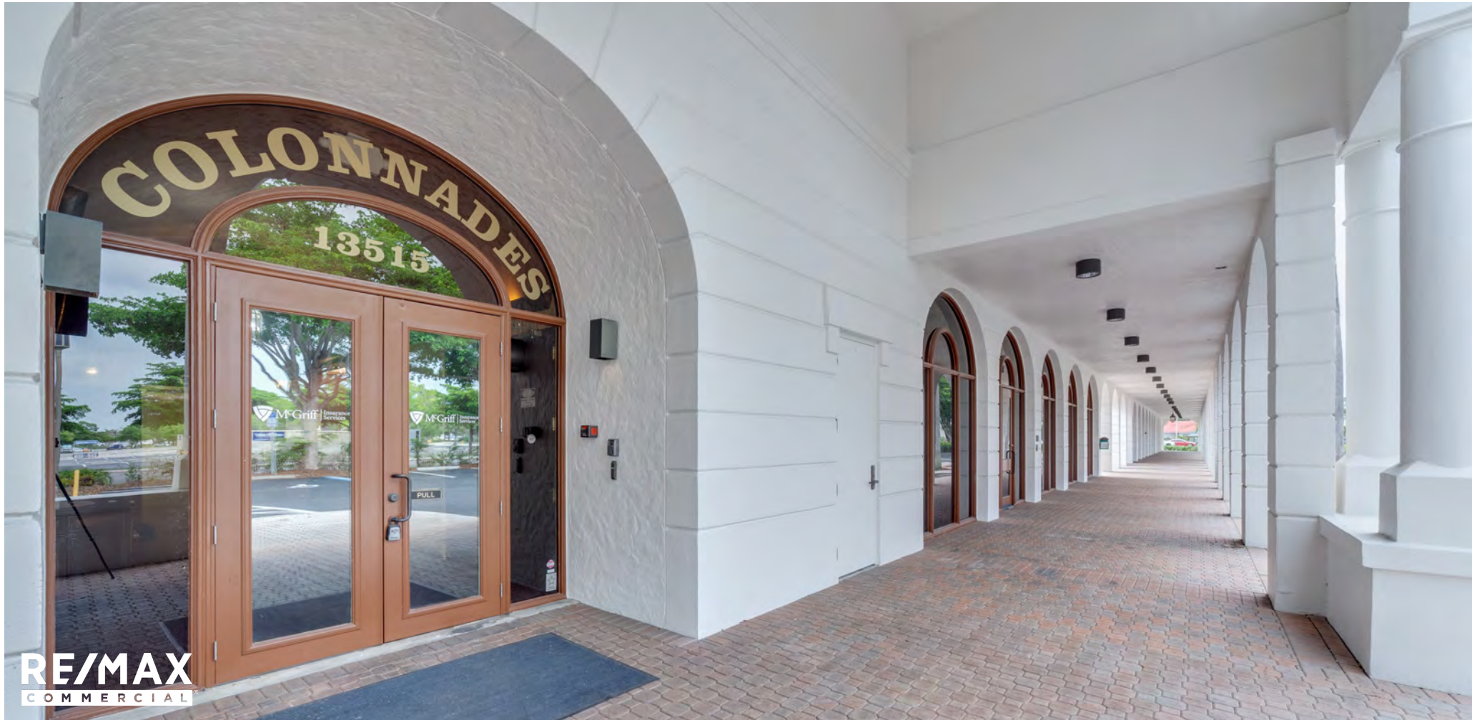
13515 Bell Tower Dr. | Main Entrance
