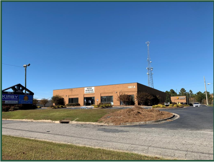
Building A Front
