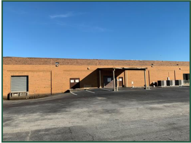
Building A Side with Roll-Up Door
