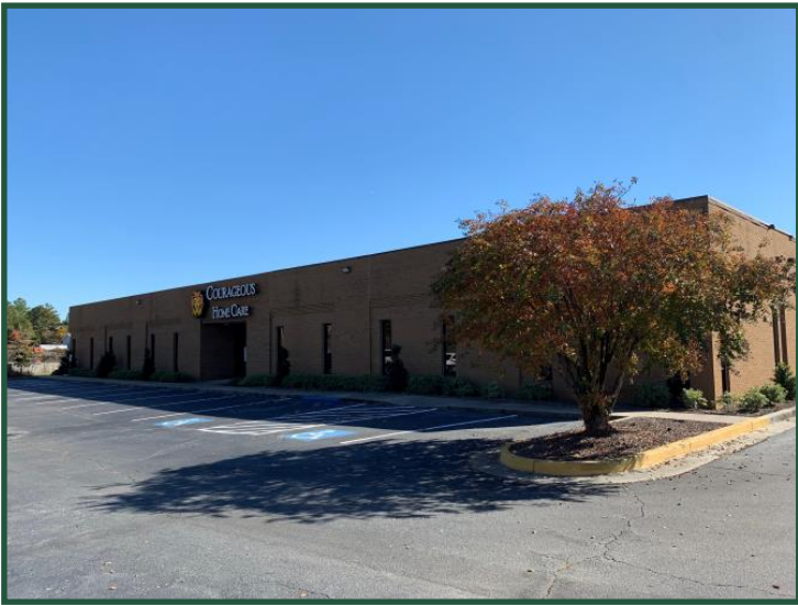
Building B Front
